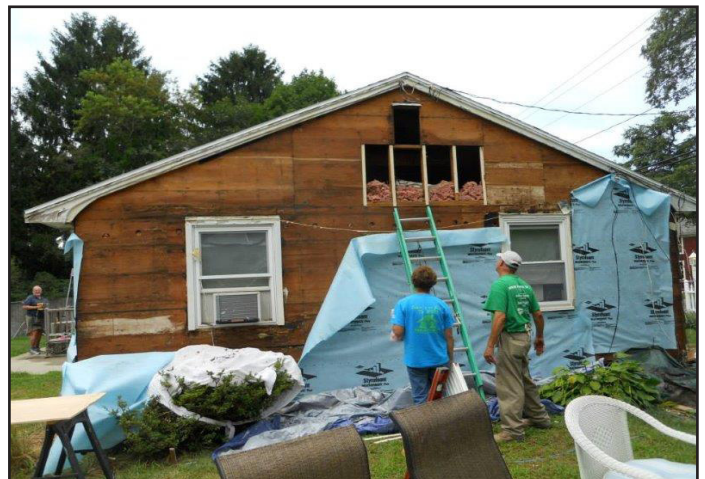
Replacing the boards.
