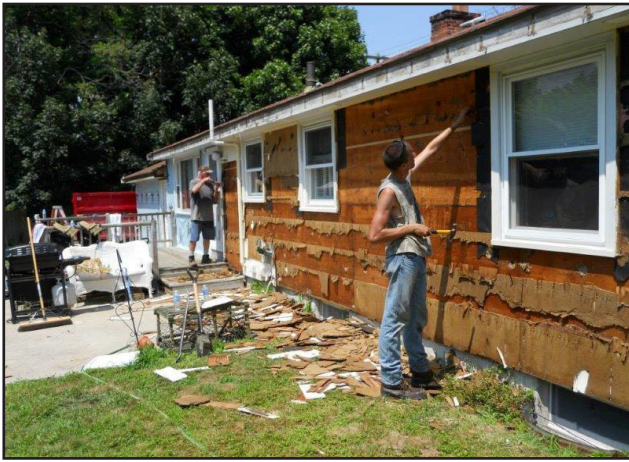
Finishing taking down the siding.
