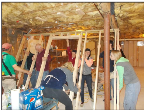
Volunteers putting up a wall at Bethany's home.
