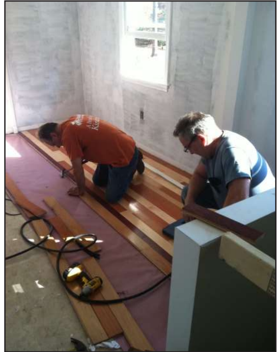
Construction crew putting new wood flooring into the home.
